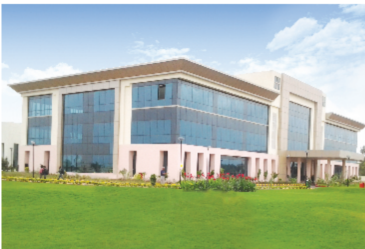
Switchgear Factory, Vadodara
