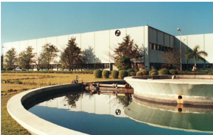
Switchgear Factory, Ahmednagar
