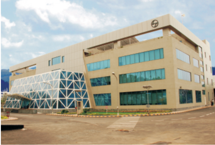
Switchgear Factory, Navi Mumbai
